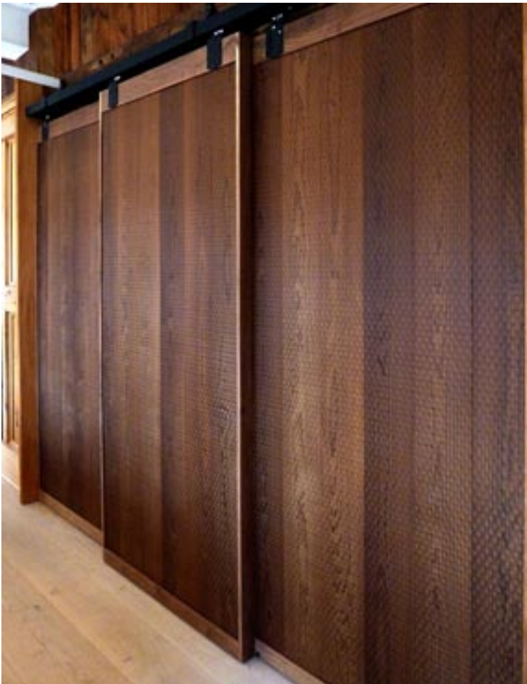
Barn door installation at the Mafi showroom in NYC
